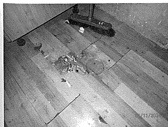
Detail podlahy kuchyne
